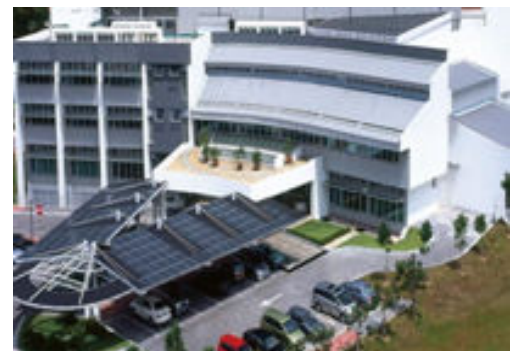
The Green Energy Office in Selangor
